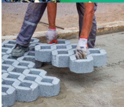
Figure 2.40 New products have been developed that allow water to move through instead of contributing to run-off. This allows the water to be absorbed into the soil and join the groundwater.
